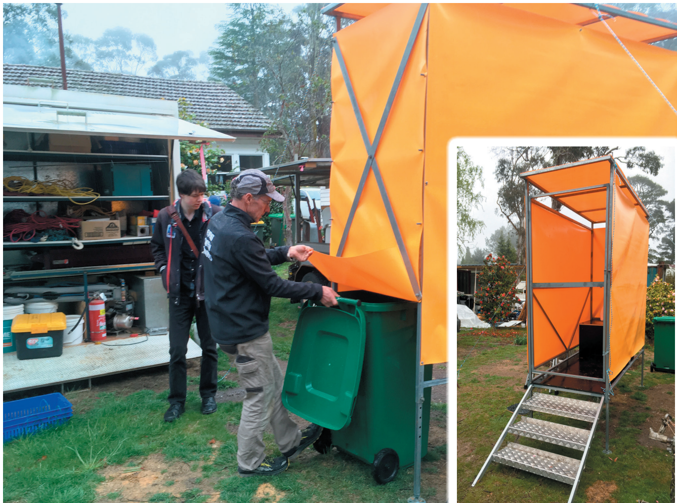
Lucas placing a wheelie bin under a composting toilet
